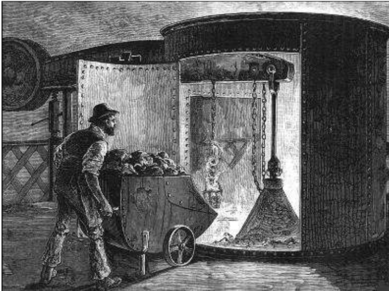
Charging a blast furnace.
